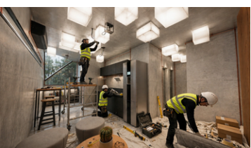
FIXTURE/ LIGHTS INSTALLATION
